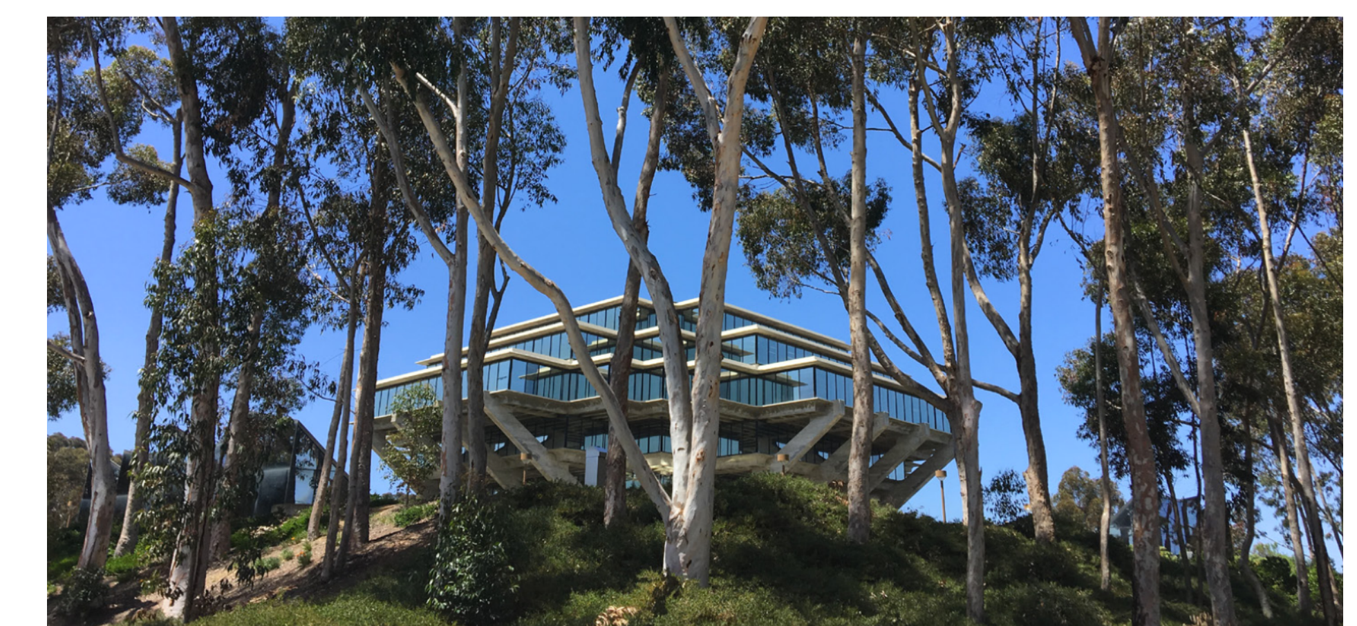
Urban Forest next to Geisel Library (Source: UCSD 2018 Long Range Development Plan)
